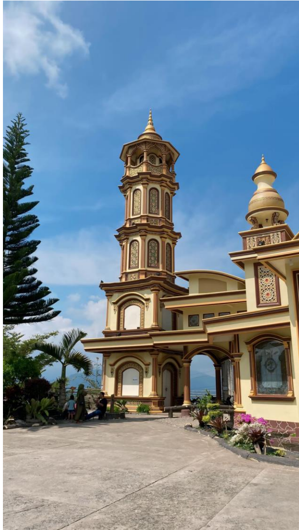
DOKUMENTASI TAMPAK SAMPING MASJID JAMI' AMINATUL JANNAH
